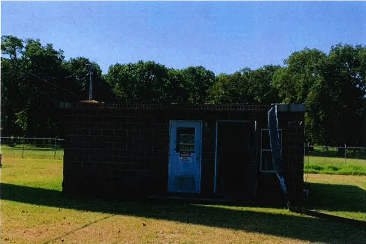
Photos of Pumphouse Roof (Taken August 29, 2020 by Clyde Woods)
